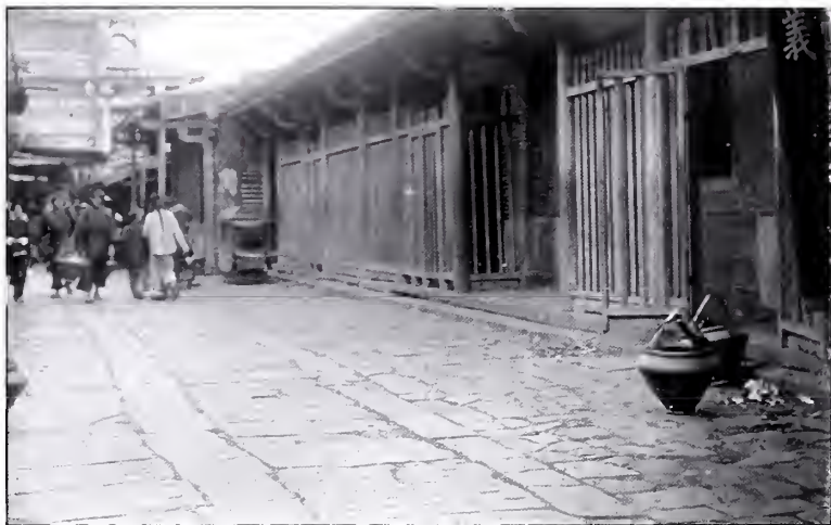
SOUTH STREET, CHINCHEW. The wooden rails are in front of the South Street Church premises. The entrance to the church is through the big gap. The nearer gap leads into our Book Shop.
